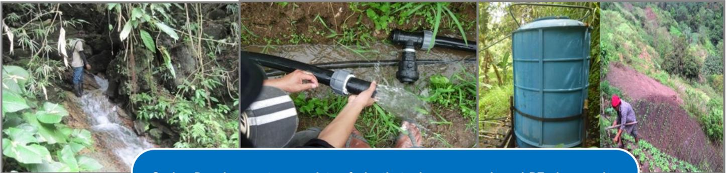
Spring Development – consists of plastic tank as reservoir and PE pipes as its delivery and distribution lines which is tapped from a high elevated body of water such as spring, creeks and the likes. This project will irrigate upland vegetables of at least one hectare. There were seven systems constructed/installed regionwide to expand the production areas for vegetable production.
